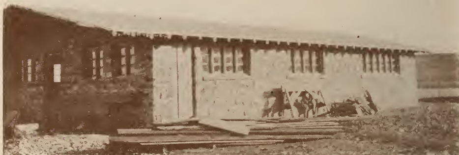
ONE UNIT BUILDING, SAINT MICHAEL'S MISSION, WIND RIVER
